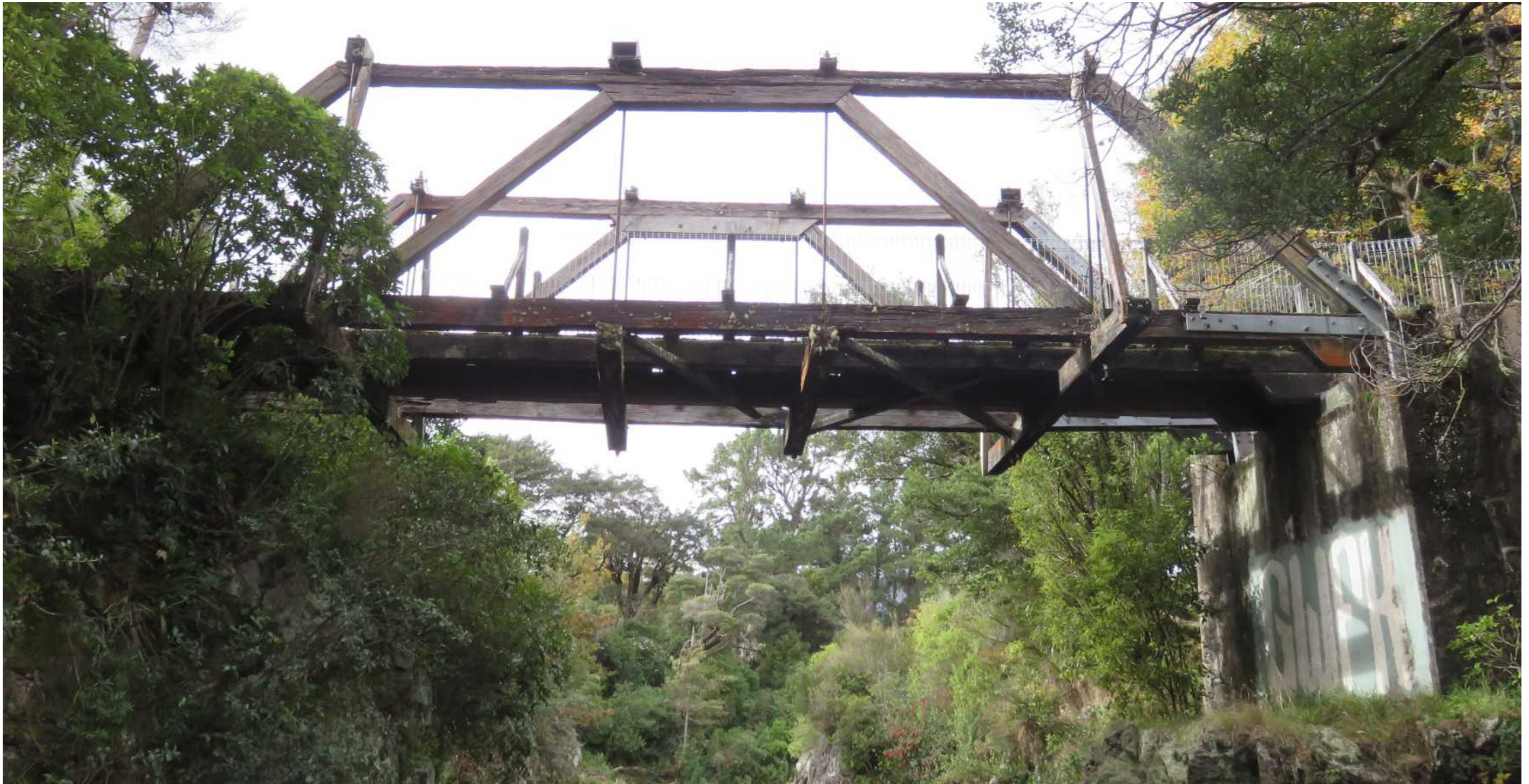
Illustration 42: Beechwood Lane facing east to bridge (22 nd May 2020).
