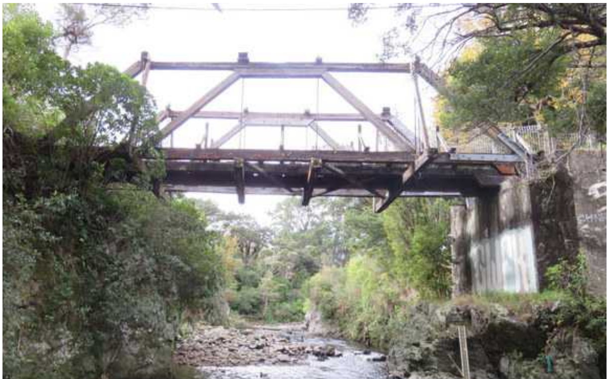
Illustration 20: Basic bridge structure (22 nd May 2020).
