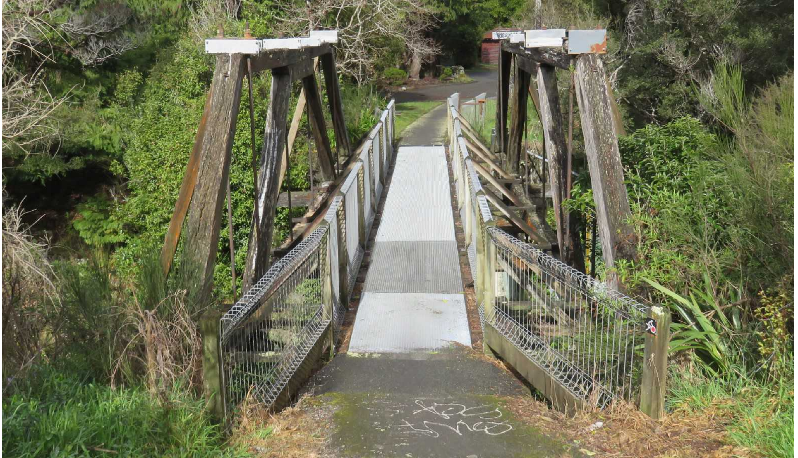
Illustration 44: Beechwood Lane bridge facing south from close to SH2 (22 nd August 2019).
