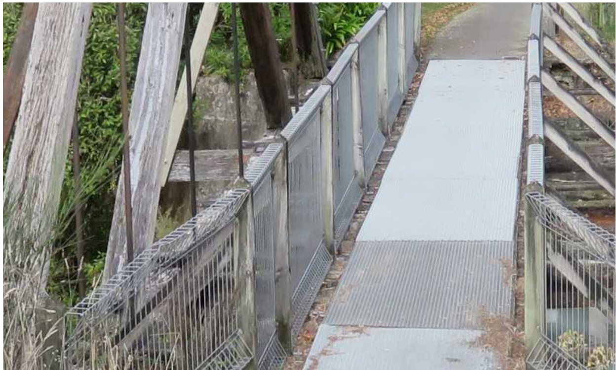
Illustration 36: Modern safety railing and deck cover (22 nd May 2020).
