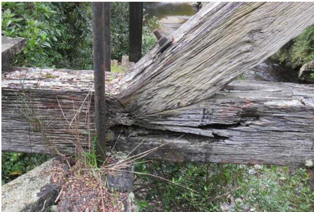
Illustration 22: End post heel joint into bottom chord (north-west end- 22 nd May 2020).
