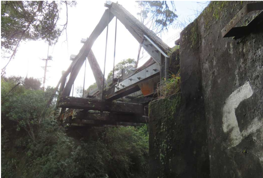
Illustration 31: Concrete abutment at south end looking towards northern end (22 nd August 2019).
