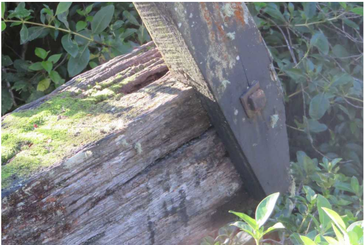
Illustration 26: Recessed butress timber secured to end of floor beam (9 th June 2020).
