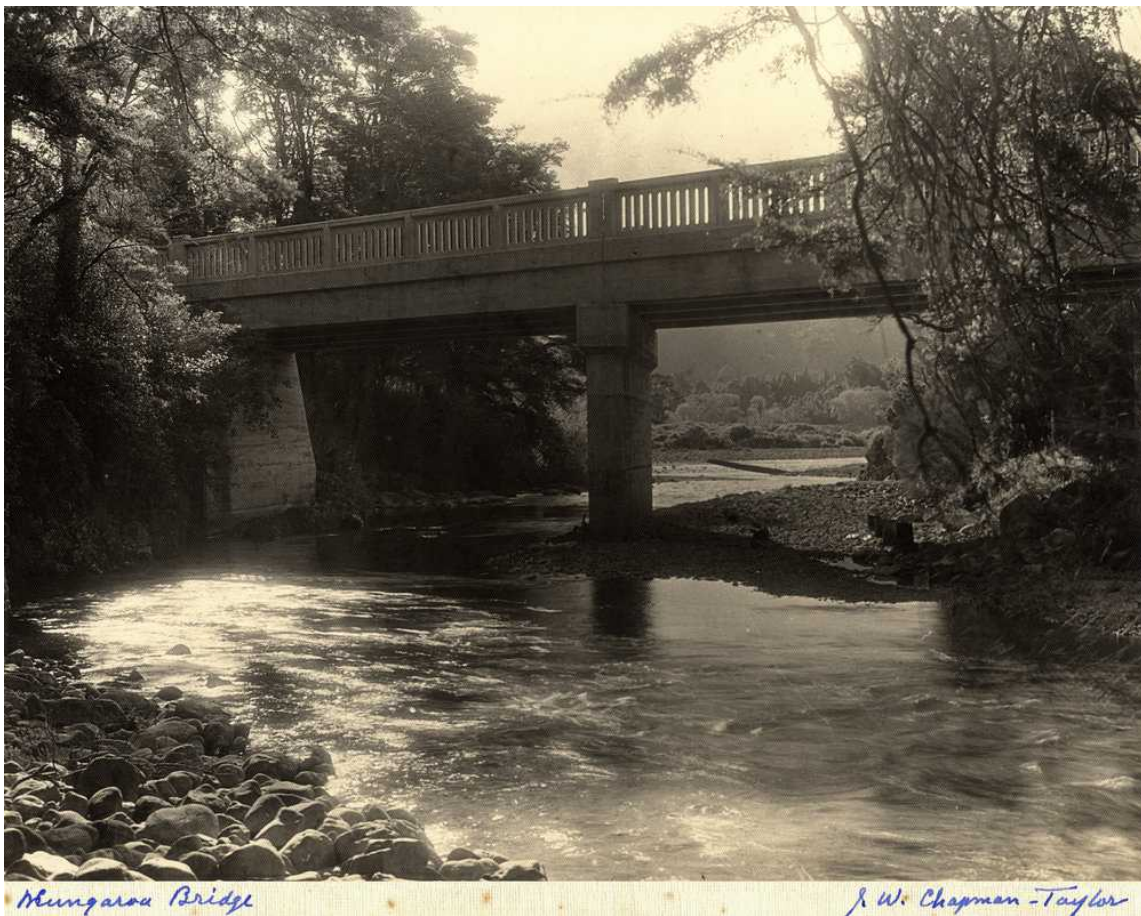
Illustration 16: Mangaroa River bridge 2, J. W. Chapman-Taylor (after 1929) (Upper Hutt City Library Heritage Collections P-49-3-2-20).
