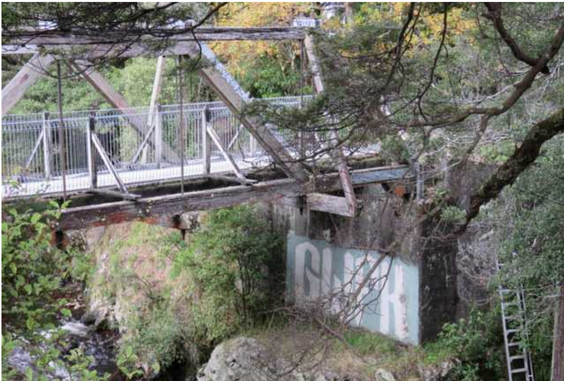
Illustration 29: Concrete abutment south end from north bank (22 nd May 2020).
