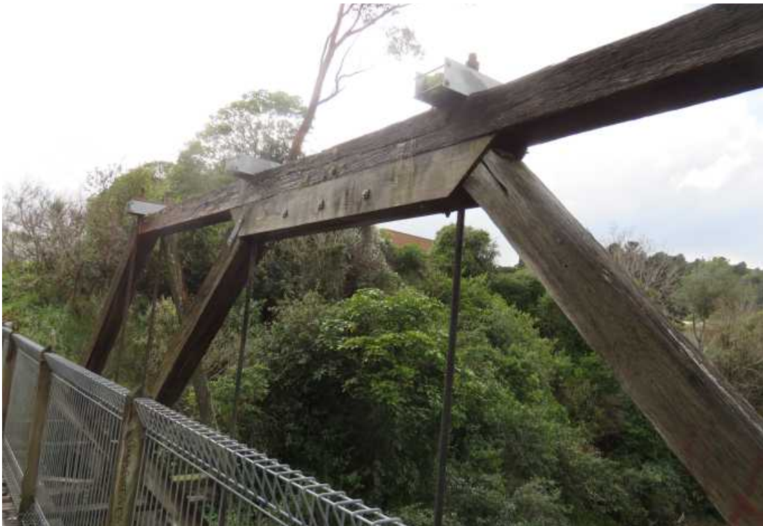
Illustration 33: Replacement pine timber transom (22 nd August 2019).
