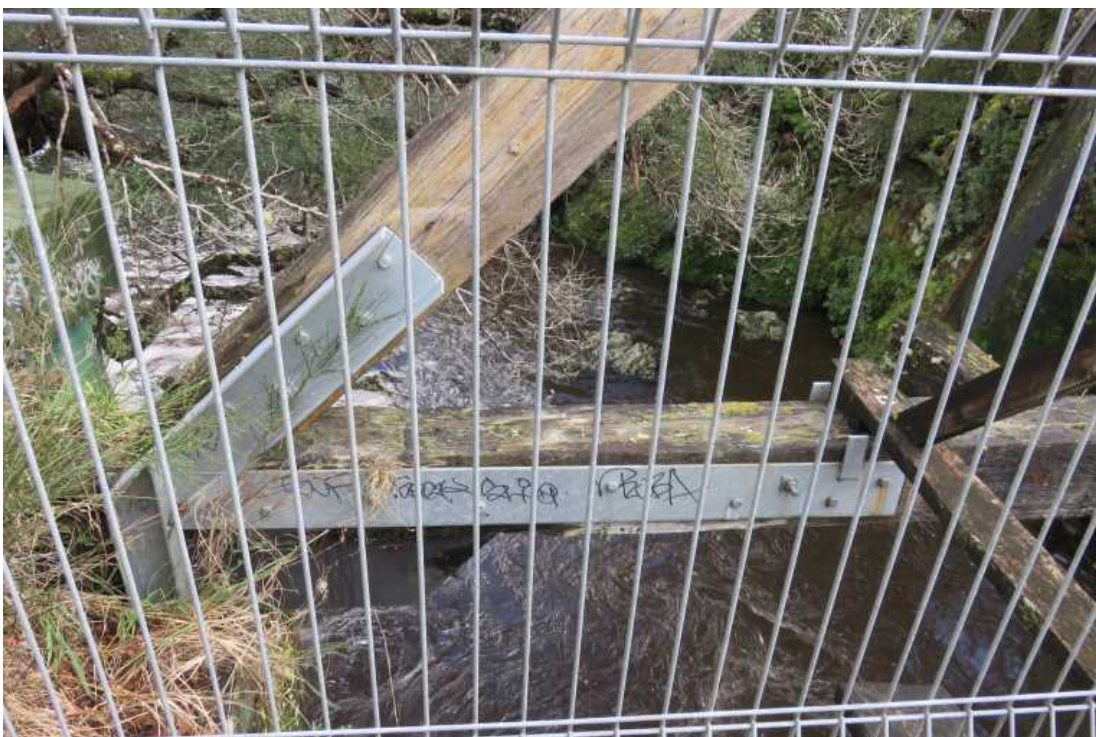
Illustration 34: Metal plates bolted to bottom chord (22 nd August 2019).
