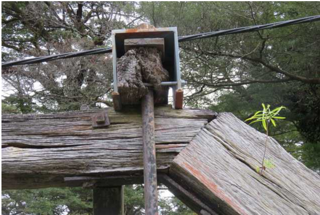
Illustration 35: Metal cap over turnbuckle timber block (9 th June 2020).
