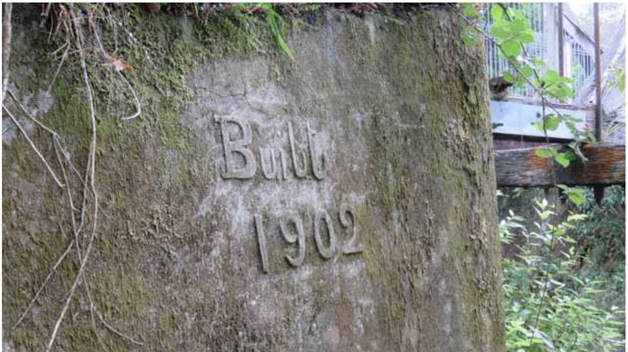
Illustration 28: Building (1902) date on concrete abutment south end (22 nd May 2020).
